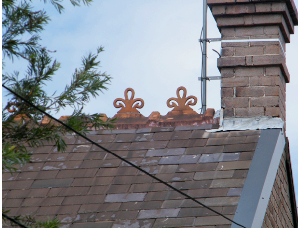
Figure 11.56. A finely detailed terracotta ridge capping to a slate roof can be overlooked in such a complex area, but adds integrity and aesthetic value to both the property and the streetscape as a whole.
